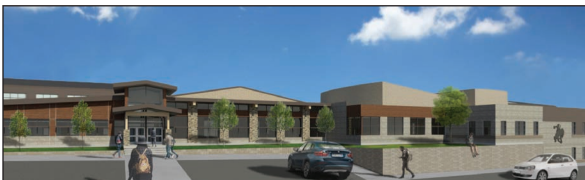
Construction will be completed in two phases over 18 months, with much of it taking place during the school year when students are on campus.
